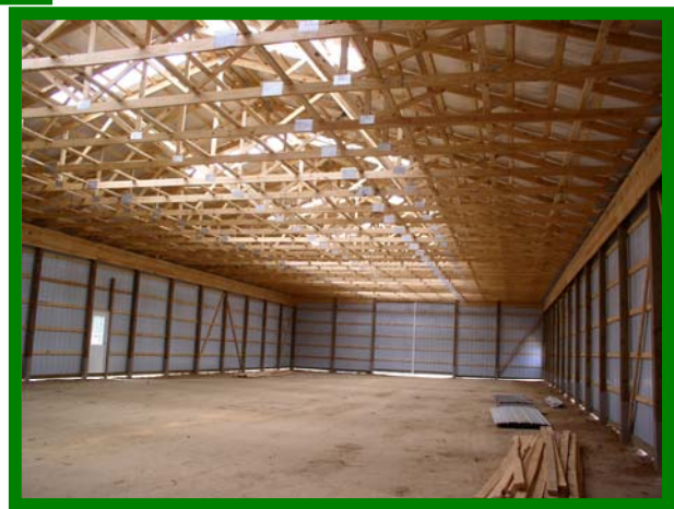
Farm Museum Under Construction
